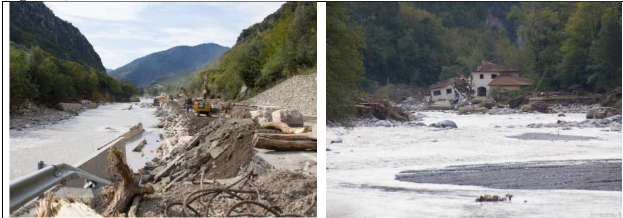
Figure 11: Road access to the south of Breil-sur-Roya are destroyed, while a temporary unpaved road is being created (left picture). A house has been cut in half by the Roya floods (right picture).
